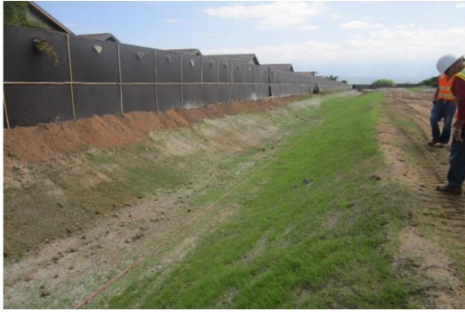
Grass-lined channel in a construction area. Credit: Anthony D'Angelo for USEPA, 2017
