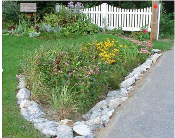
A rain garden is a bowl-shaped garden designed to capture and absorb stormwater.
